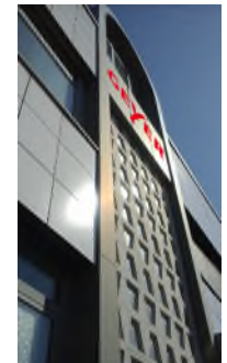
Geyer Global Headquarters Design and Test Center Munich - Germany
