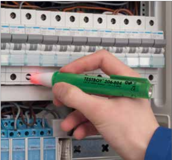
Testboy illuminates with voltage present
