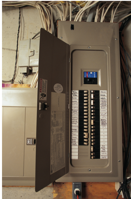
Small power distribution and circuit breaker panel suitable for incorporation of energy measuring module.
